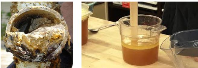
FOG and Scum typically have a specific gravity of  $<1$ , causing it to decant from water and float on the surface. If allowed, this decanting will form large floating mats that will accumulate over time. The simple pumping operation of a wet well will also create this mat. As the pump cycles from on/off, it is merely dewatering the from under the floating mat. This mat will thicken with each pumping cycle and reduce the liquid volume of the wet well.
