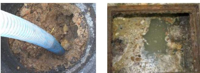
When pumping wastewater with FOG and Scum, it is important to keep things turbulent and mixed within the wet well. It is also important that the pump head (volute/impeller) be submerged in the wet well. FOG/Scum has been known to plug suction lines, restricting the flow to dry well pumps and causing pre-mature pump failure.
