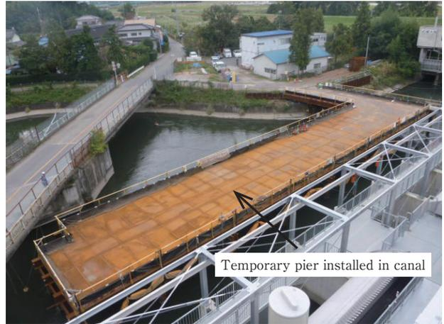
Temporary pier installed in canal
