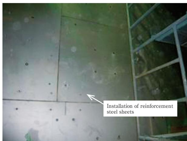
**Fig. 9** Civil engineering work for seismic retrofitting (Pump sump section)
