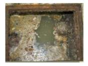
When pumping wastewater with FOG and Scum, it is important to keep things turbulent and mixed within the wet well. It is also important that the pump head (volute/impeller) be submerged in the wet well. FOG/Scum has been known to plug suction lines, restricting the flow to dry well pumps and causing pre-mature pump failure.
