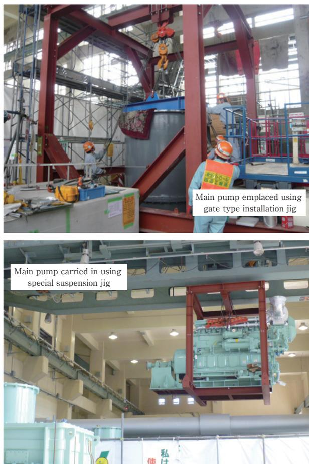
**Fig. 10** Carrying-in and emplacement of main pump using installation and suspension jigs
