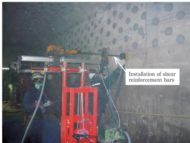
Installation of shear reinforcement bars
